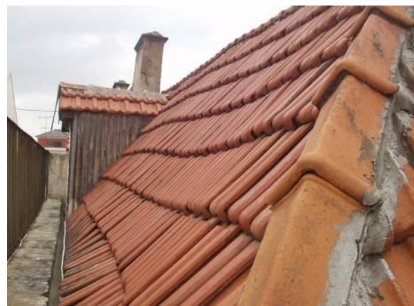
(b) Cobertura mansarda
